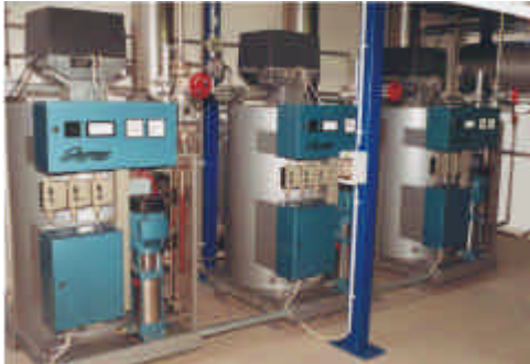
Jumag steam generator three-fold unit 960 kg/h steam generating capacity Saxonia Medical, Radeberg
