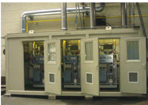
Jumag Container three-fold unit Steam generating capacity 960 kg/h BEWAG, Berlin
