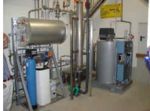
Jumag steam generator DG320 Complete with water purification Weingut Anselmann, Edesheim
