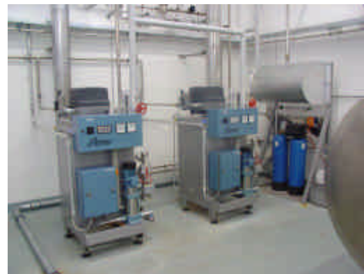
Jumag steam generator two-fold unit with 2 x 160 kg/h Schwan-Stabilo, Heroldsberg
