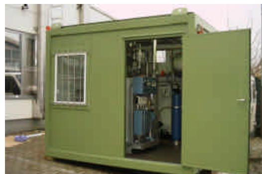
Jumag Container steam generating unit Steam generating capacity 320 kg/h RAG-Österreich
